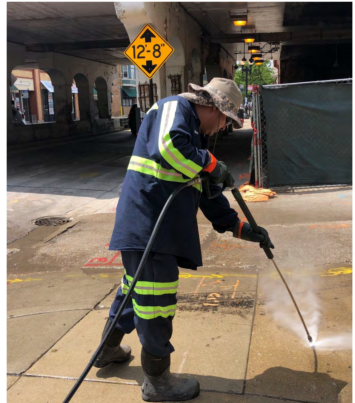
SIDEWALK POWER WASH
