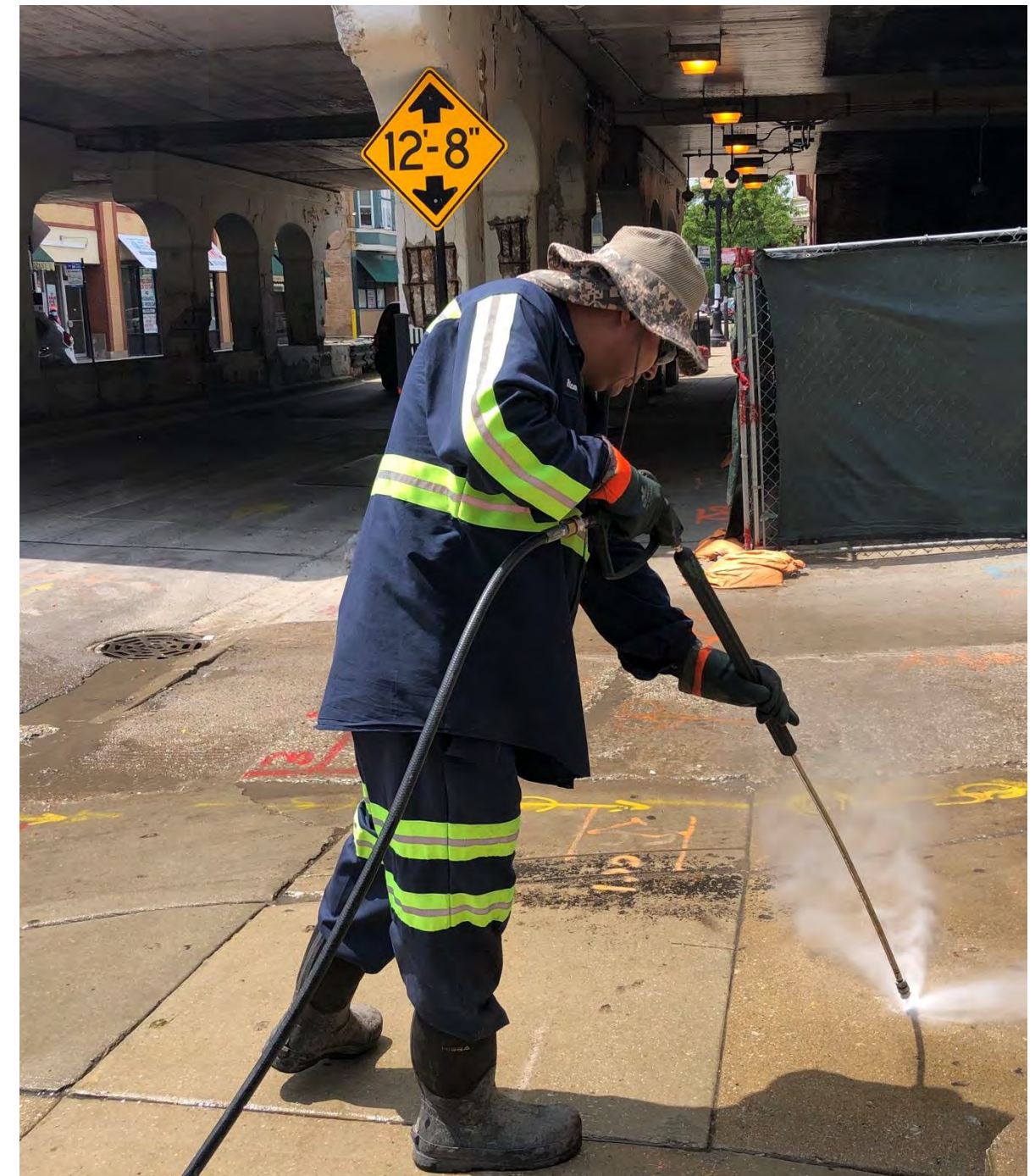
SIDEWALK POWER WASH
