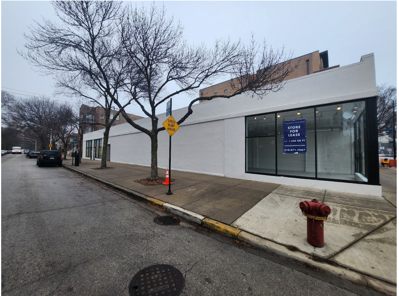
Exhibit 1: South facing wall at 6116-18 N. Broadway
